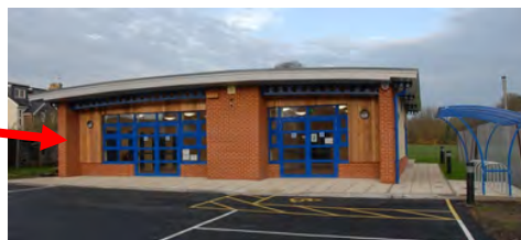
Dunton Green Pavilion RECREATION GROUND, LONDON ROAD
